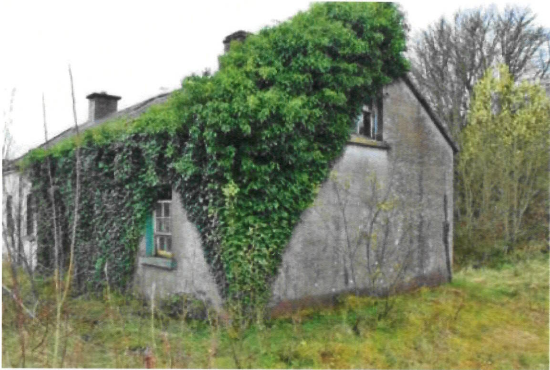
Front Elevation before start of works
