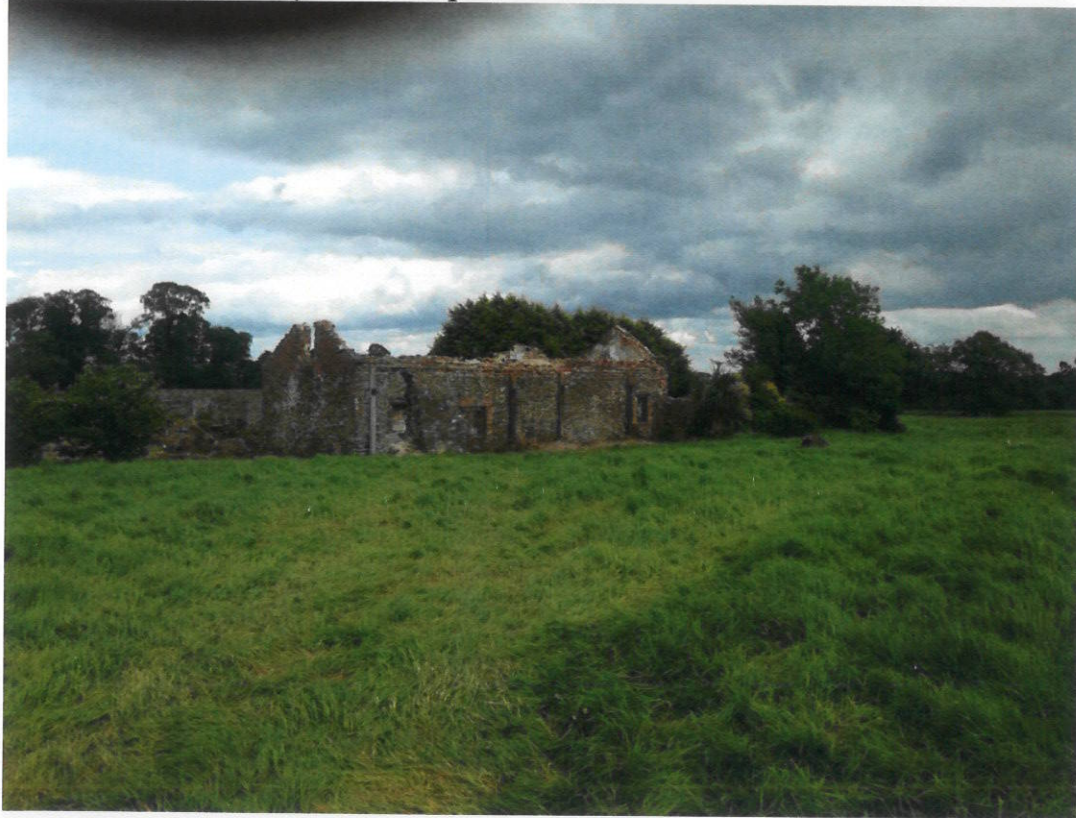
Rear Elevation – ivy roof and plaster removed
