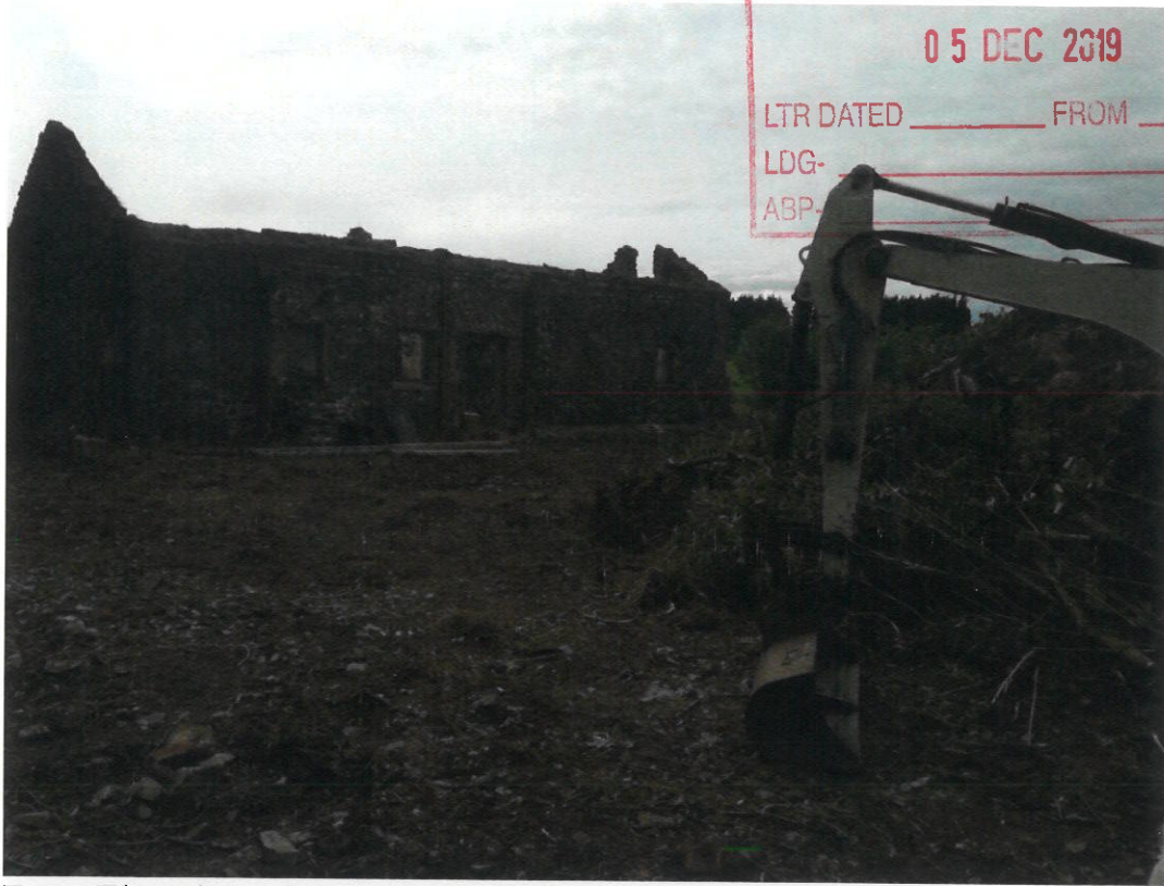
Front Elevation – ivy roof and plaster removed
